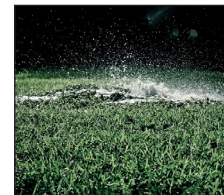
Malfunctioning septic systems
