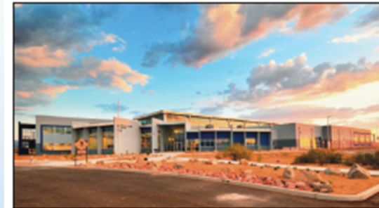
Orenco's AdvanTex ® Wastewater Treatment System was installed at the Andriada Politechnico Palano High school campus near Tucson. (Story on back)
