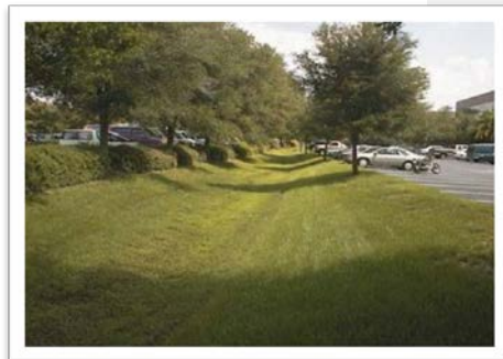
Figure 41. Dry swale. Photo by Virginia DCR Stormwater Design Specification Manual, No. 10.
