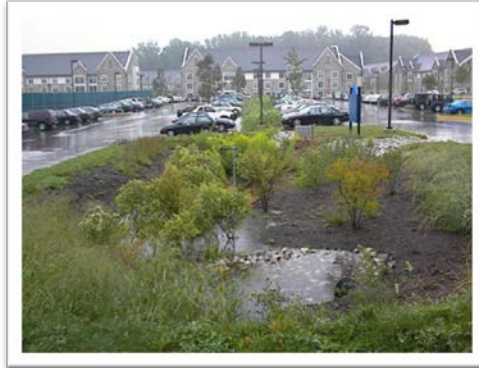
Figure 4. Biofiltration/Rain Garden slows storm water runoff from parking lots. Photo by Temple-Villanova Sustainable Stormwater
