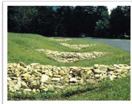
Figure 22. Rock berm installations on dry drainage area. Photo by Lake Superior Streams: Grassed Swales.
