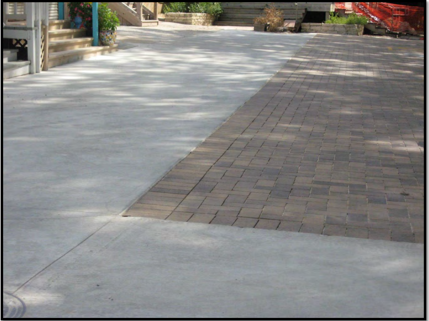
Pavers and Concrete Edge Interface
