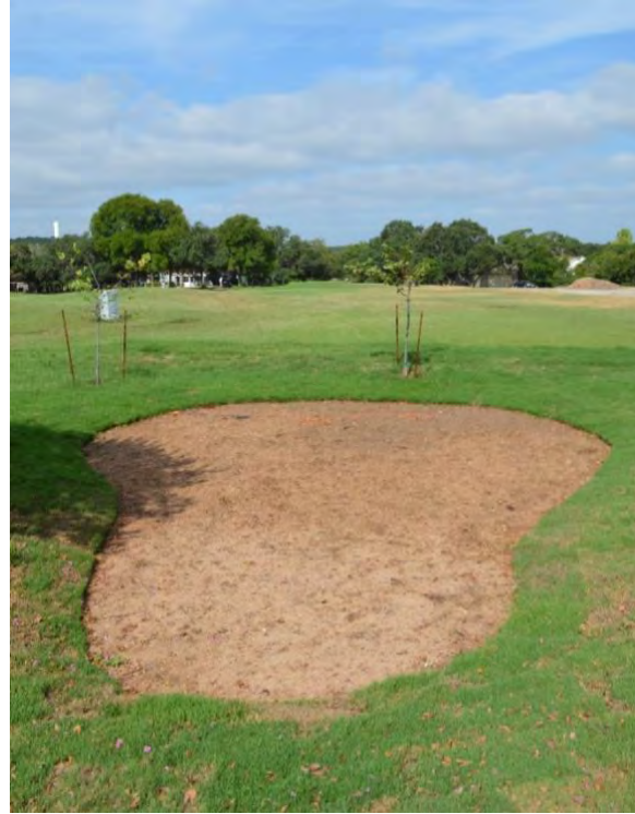
Figure 6. Rain garden at Woodcreek Community Golf Course just after completion, pre-plant
