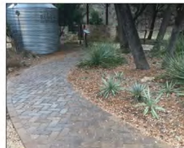
Permeable paver sidewalk at Blue Hole Regional Park
