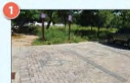
ADA Parking Spots
