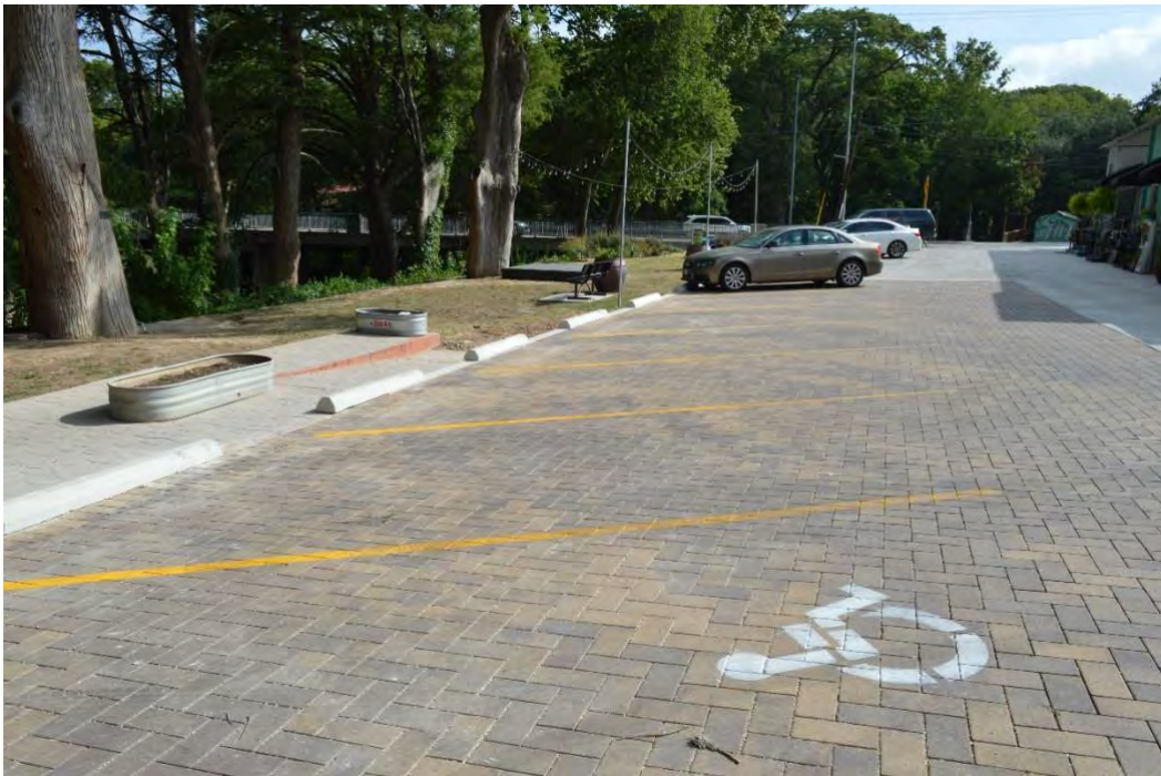
Figure 5. Permeable Paver parking lot in Downtown Wimberley
